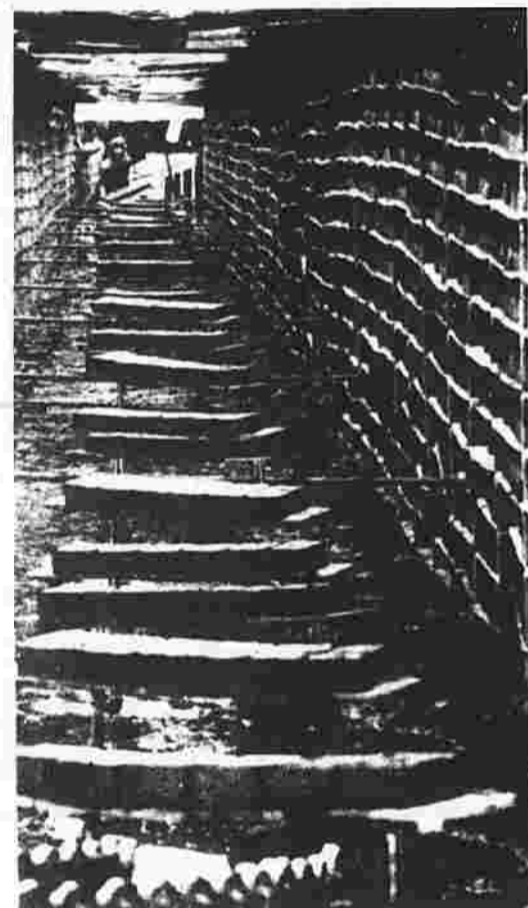
Wire conveyor carries fresh bricks to drying racks to air dry.
