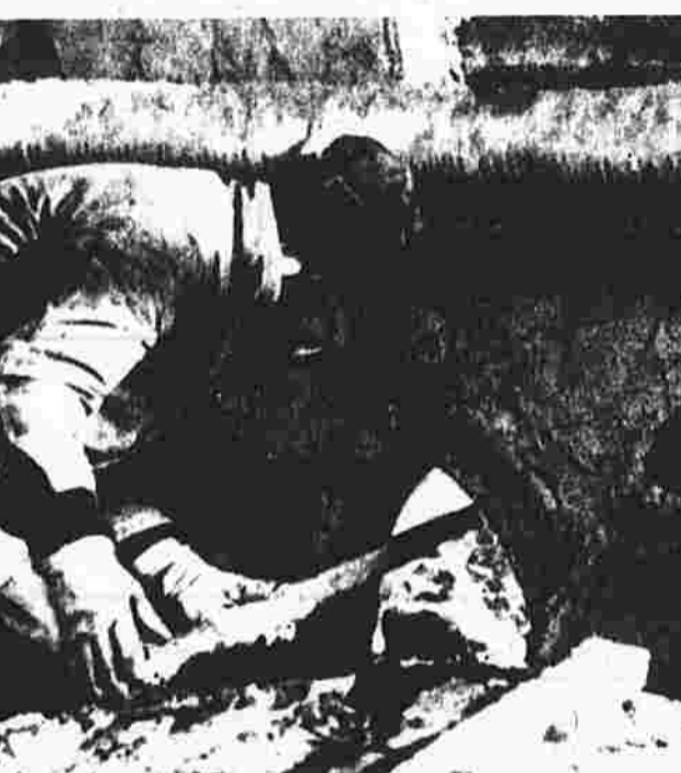
After the bricks are stacked and covered with mud to form the kiln, pine logs are used in the week-long firing process.
